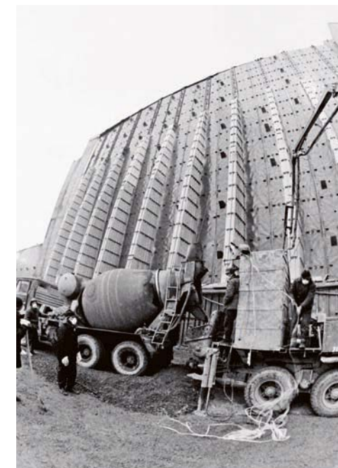
NON-STOP EMERGENCY DEPLOYMENT In the months after the meltdown, Putzmeister pumps operated around the clock
