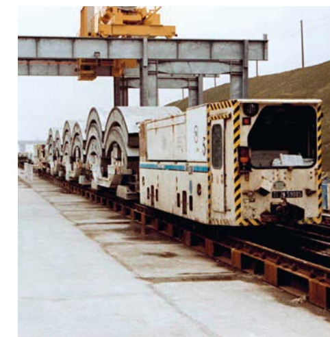
ON THEIR WAY TO THE CONSTRUCTION SITE Transportation of the reinforced concrete rings from which the tunnel pipes were produced. Great precision was required when placing the concrete.
