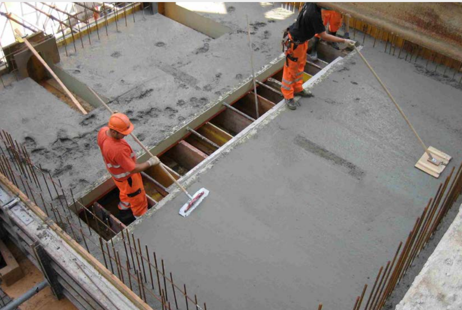
Construction of a concrete reception bunker
