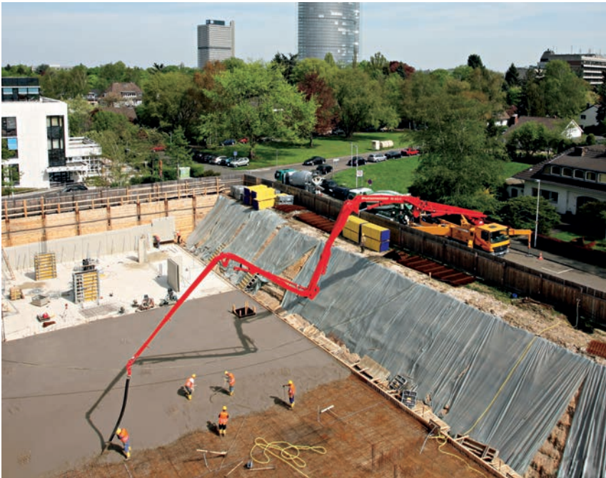
Abb. 1: Putzmeister Autobetonpumpe M 42-5 in Bonn
