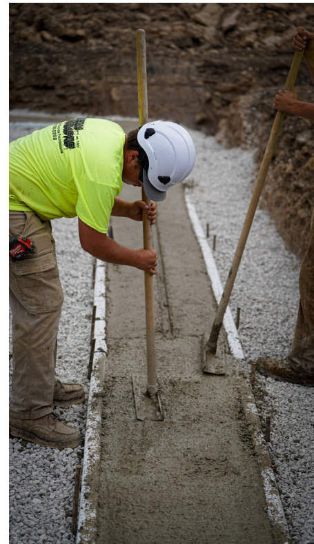
A high school student learns how to smooth out the wet concrete of the home’s foundation
